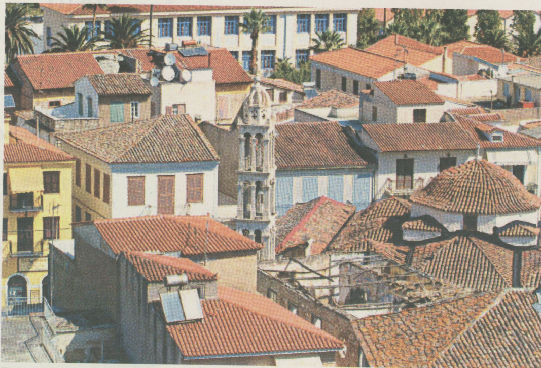
They might be picturesque and quaint, but how would these old buildings in Nafplio score in the new energy-rating procedure?
